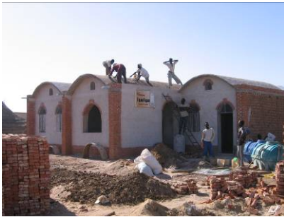
Figure 9: construction in process ©Practical Action
