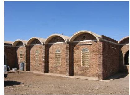
Figure 11: finalized – exterior view ©Practical Action
