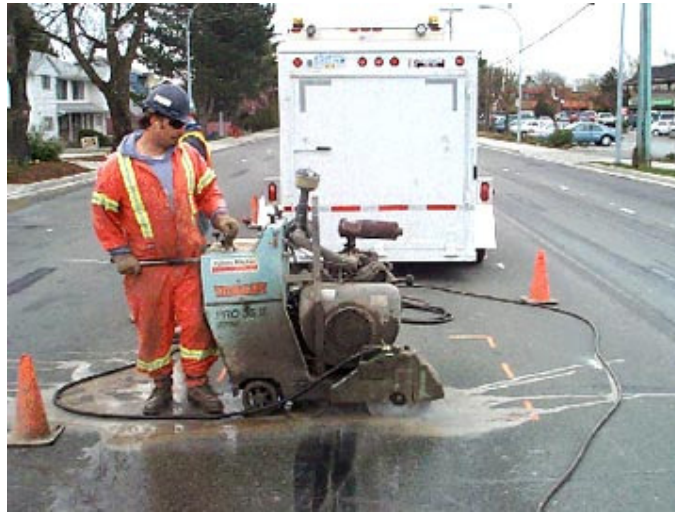
Exhibit 1-2 – Induction Based Traffic Loop Installation 5
